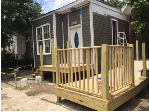
Work in process on the Baham's new ramp
