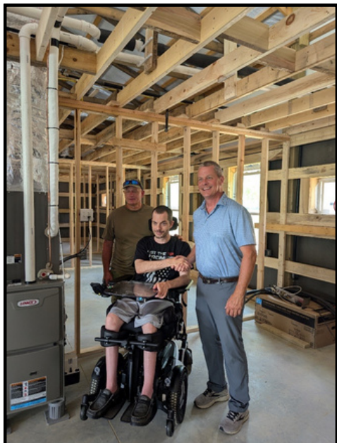
John Milligan with Mike Thorne (installing contractor).
