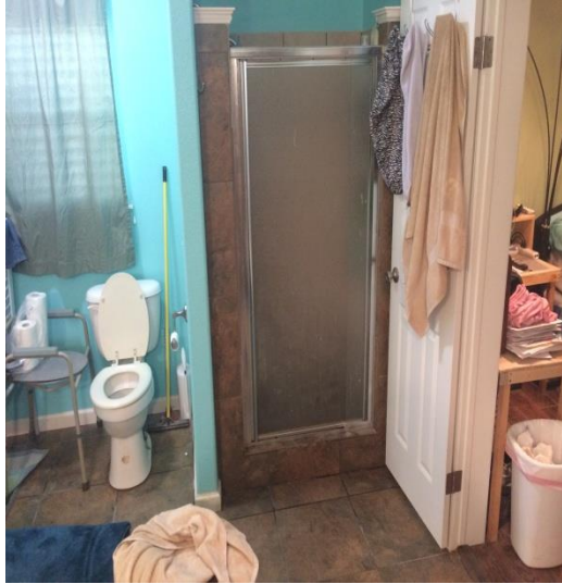
Bathroom before remodel
